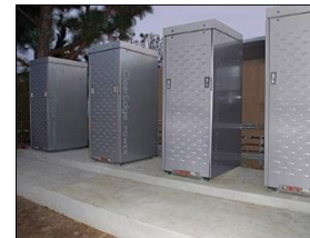
ClearEdge Power (OR) 5 KW Fuel cell mCHP
