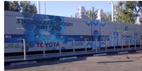
Oct 2012, Ballard 1.1 MW ClearGen fuel cell operated at Toyota Headquarter in Torrance, California
