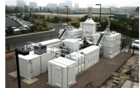
FuelCell Energy DFC 300 2.8 MW MCFC
