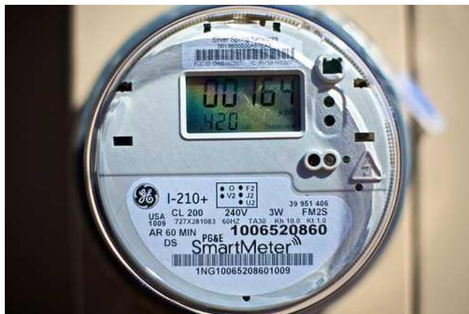
**Smart meters** can be used to collect 15-min interval (whole building) electricity data.
