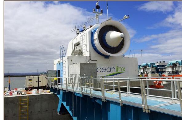
Oscillating water column: Oceanlinx
